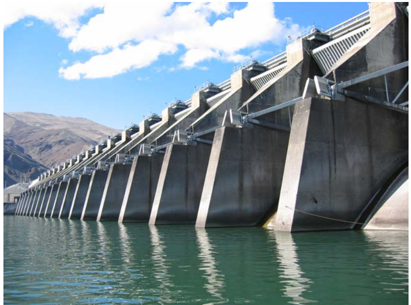
Priest Rapids Dam Spillway Repairs
